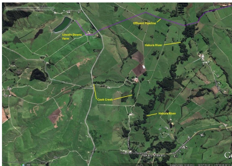
FIGURE 13: Location of Cook Creek, the Effluent Pipeline and the Hakaru River - Source Google Earth
