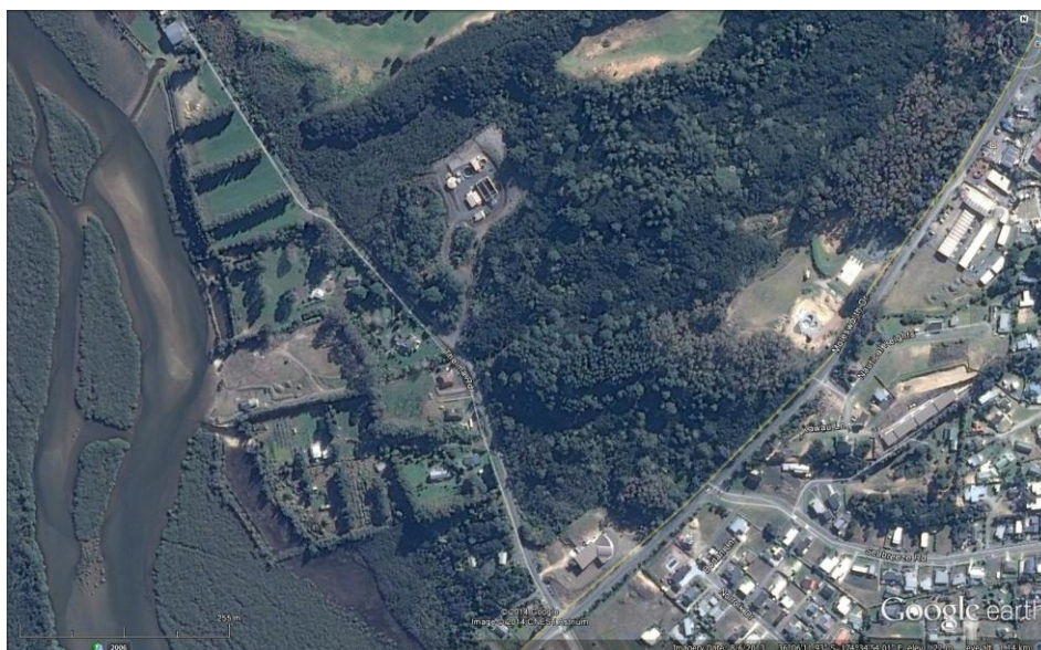
FIGURE 4: Mangawhai Wastewater Treatment Plant off Thelma Road (top centre) - Source: Google Earth
