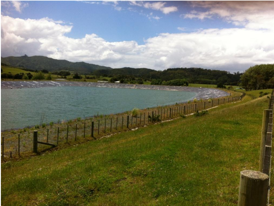
FIGURE 5: Effluent Storage Lagoon, Lincoln Downs Farm - Harrison Grierson
